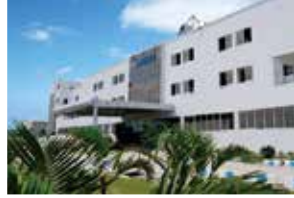
Rudrapur Plant (Green Building)
